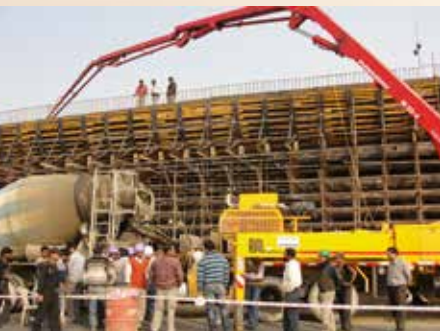
Inspection of Concreting work at Flyover Site
