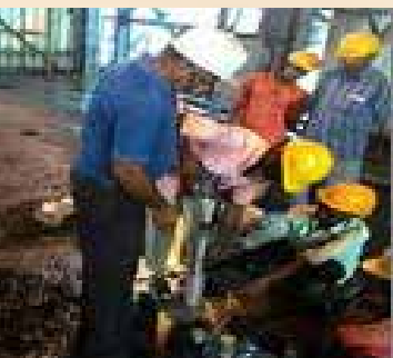
Core Extraction from Fire Damaged Structure
