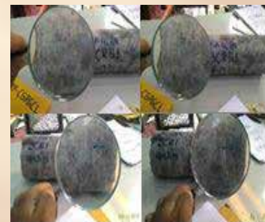
Crack width Measurement from Extracted Core
