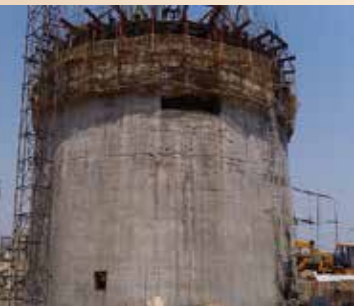
Structural Assessment of under Construction Chimney
