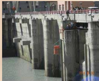
Field Investigation for Residual Life Assessment of Dam Structure
