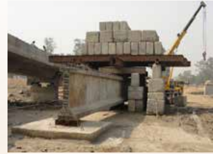
Load Test on Pretension Girder for Flyover Project
