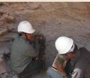
Pile Integrity Test of Prestressed Concrete Bridge
