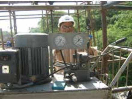
Witness of load applied during post-tensioning of Bridge Deck
