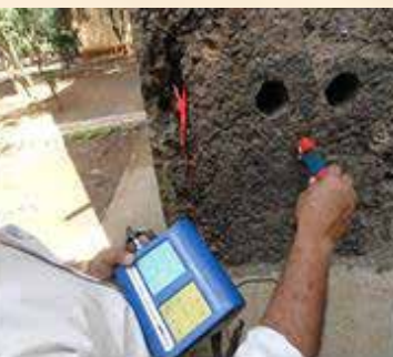
Half-cell Potential Measurement of Corrosion Damaged Structure
