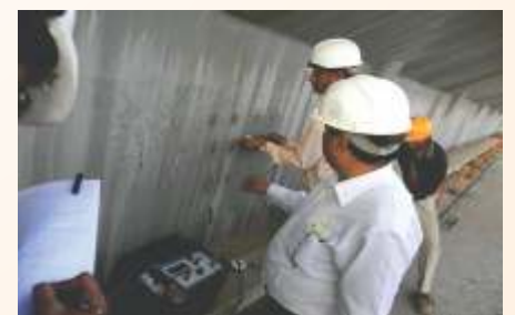
UPV test of Concrete Structure for Quality Assessment
