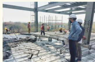
Non-Residential Buildings using Pre-Engineered Construction Technology at KG Marg and Africa Avenue, Delhi
