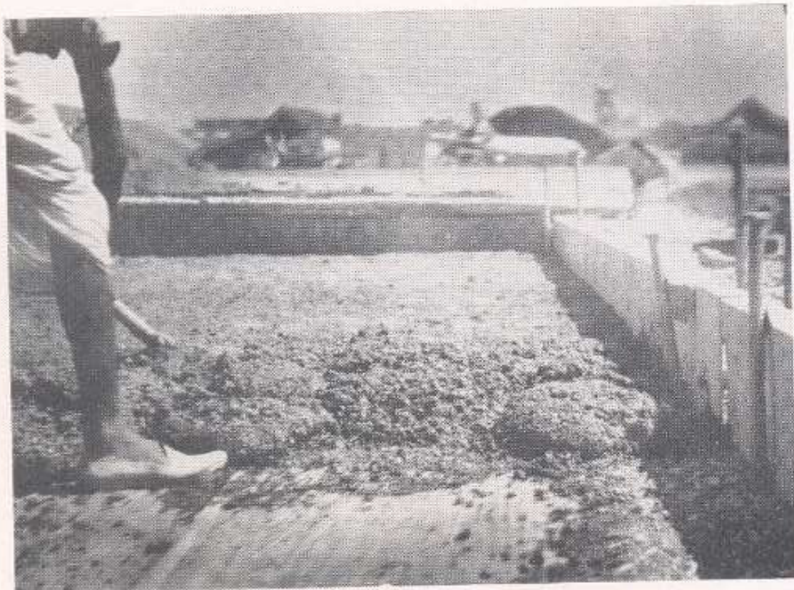
Fig 3 Compacting of SFRC with needle vibrator
