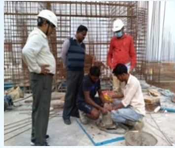
Slump test at Site
