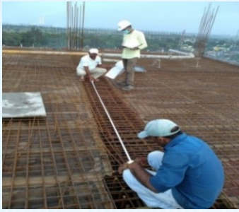
Checking of Steel Reinforcement
