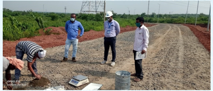
Inspection of Road Work
