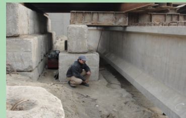
Load Test on Prestressed Concrete I Girder
