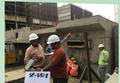
UPV test of Concrete Structure for Quality Assessment
