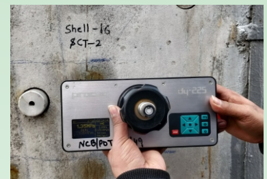
Pull-Off Test Being done to check bonding of PMM with substrate concrete
