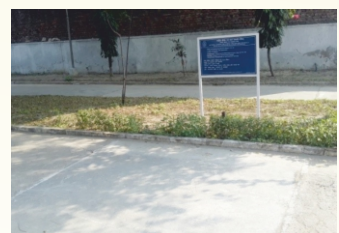
Trial Stretch made using Geopolymer Concrete
