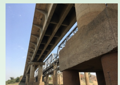
Condition Assessment of RCC Bridges
