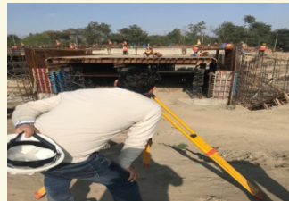
Underpasses / Tunnel works in Pragati Maidan- PWD, New Delhi
