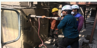
Core extraction from RCC foundation
