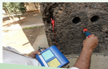
Half-cell Potential Measurement of Corrosion Damaged Structure
