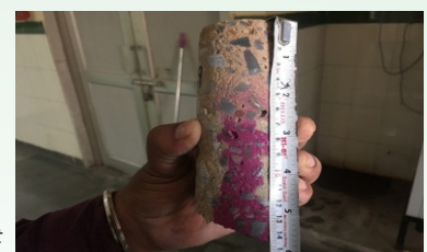
Carbonation depth being measured on freshly extracted core at site
