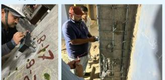
NCB Team carrying out Pull-off test on repaired columns and checking electrical continuity of installed anodes at NHAI site
