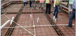
Reinforced slab structure with embedded strain gauges before concreting
